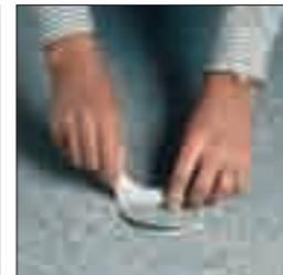
(3) Put the arm of the knife on the pivot (the smallest hole) and cut the hole.
