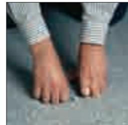
(2) Lay the vinyl over the gully and press until the pivot on the foot penetrates the vinyl.
