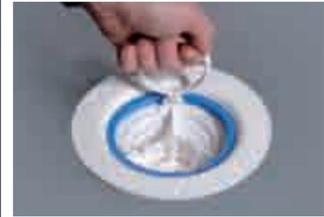
(1) Pull up the handle and lift off the water trap.
