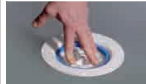
(5) Wet the rubber gasket with water and press the water trap in place
