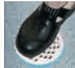
(6) Place the clamping ring in the gully with the text facing upwards. Press it down with the grating.
