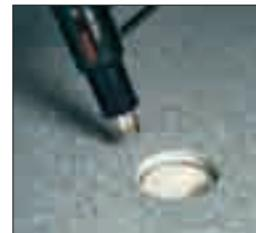
(5) Heat the vinyl. NOTE: rubber cloths shall not be heated.
